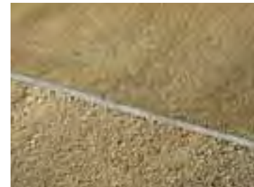
Rolled aggregate into asphalt.
