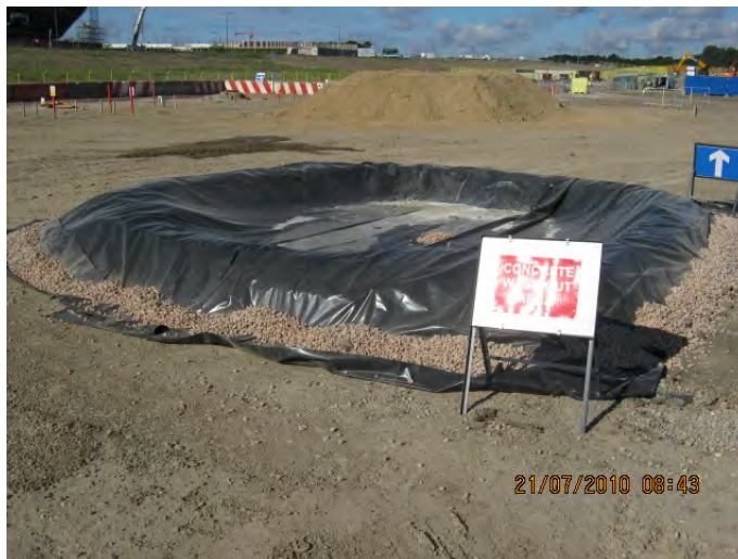
Figure 1 Example of a concrete washout facility
