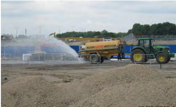
Figure 5 Example of watering haul road to suppress dust and road sweeper
