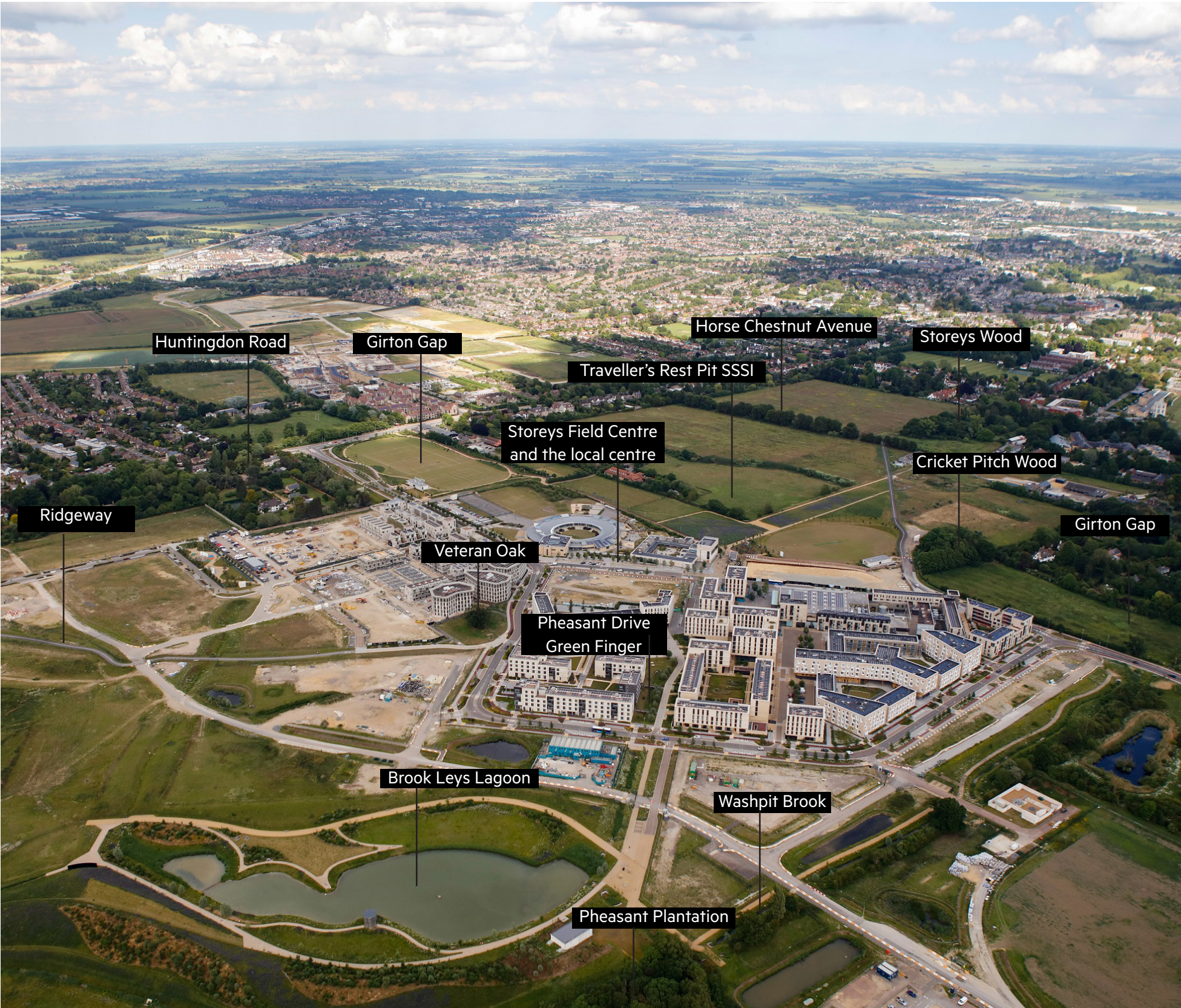
Aerial view of Eddington, Phase 1 in progress
