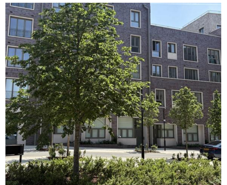
Example: Forest scale tree within open space as a marker and pivot point for circulation routes
