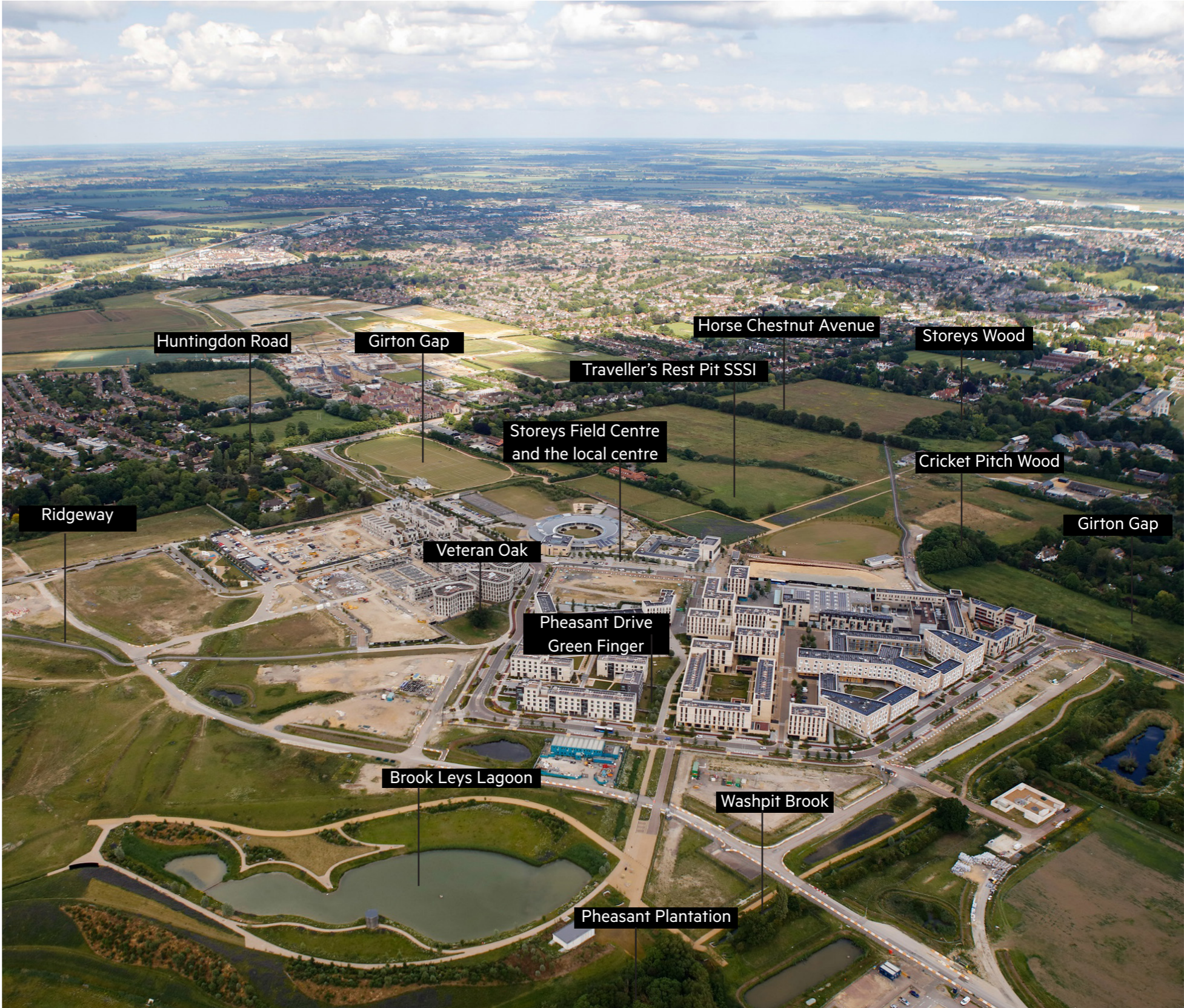
Aerial view of Eddington, Phase 1 in progress
