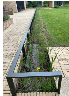
3. Well detailed small water feature as part of the SuDS strategy
