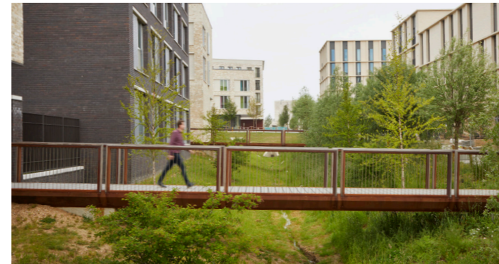
5. Bridge crossings are not the most effective and inclusive access solution
