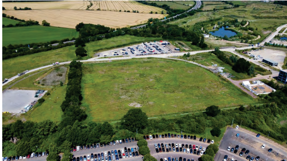
Photo A5.9: Pheasant Plantation, lagoon at Brook Leys (Zone 3c), temporary haul road and car park construction areas (Zone 5d)
